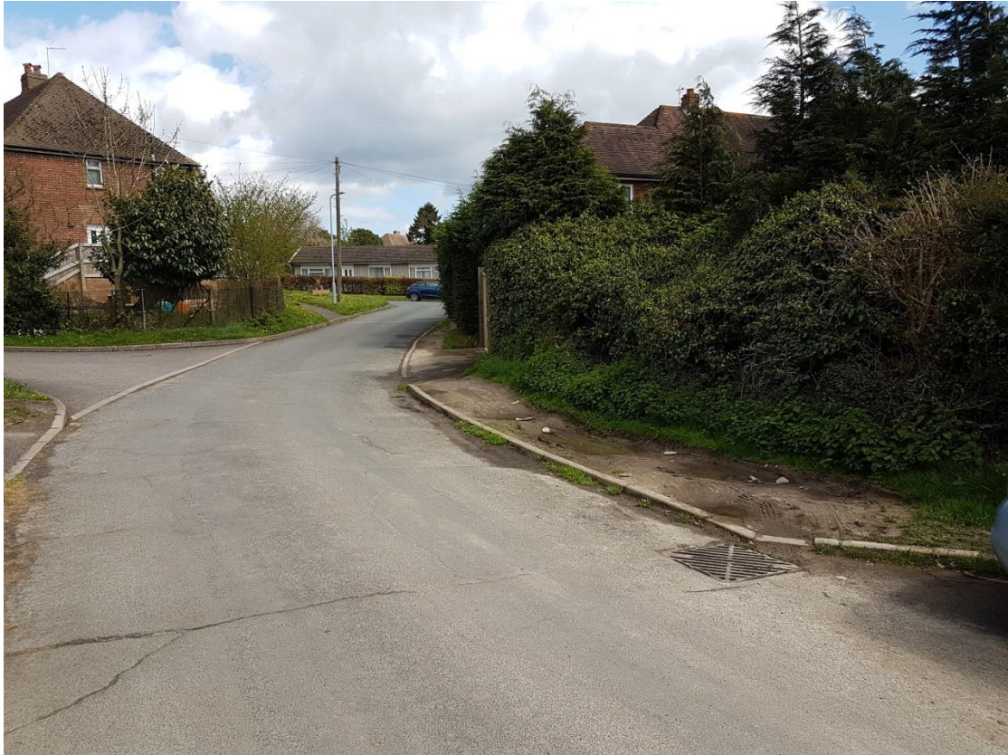
Photo 5 - evidence of verge damage due to reduced width of carriageway
